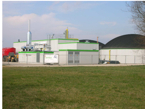
Biogasanlage in Angelbrechting
